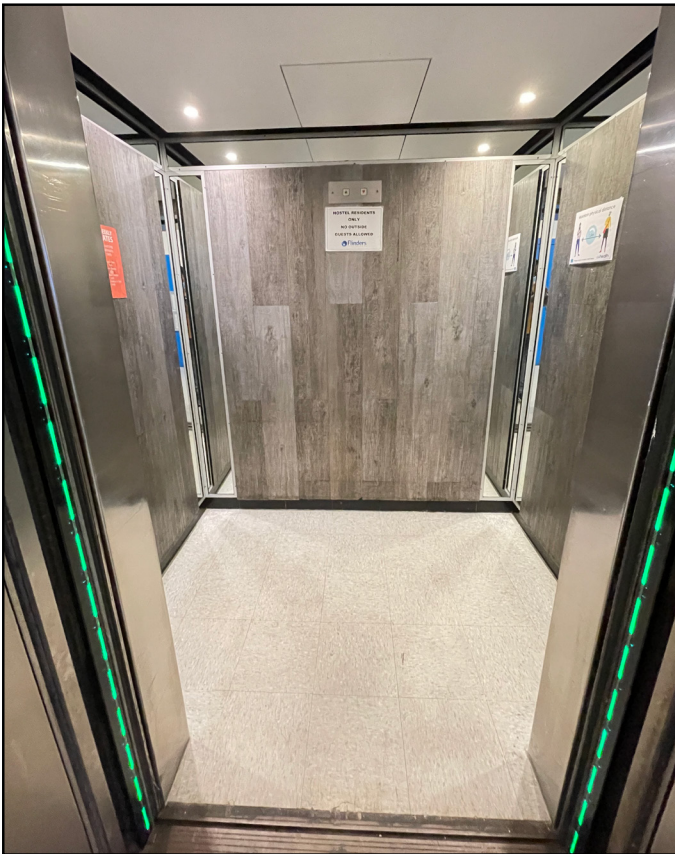
Elevator door frame Height: 2025mm Width: 1065mm
